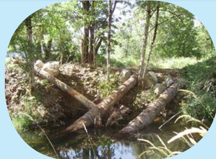
During 2009-10, six habitat structures were added in the floodplain and stream, off-channel habitat areas were created, and a 2.5 acre riparian area was restored.
